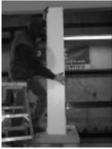
13) Screw or nail column to blocking ONLY ON THE BOTTOM . Do not attach at center or top (to allow for expansion.)
