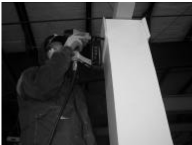
19) Option 2: Leave ¼" expansion room above cap, and pin-nail the cap to the column. Be sure pin-nails DO NOT reach the blocking inside!*
