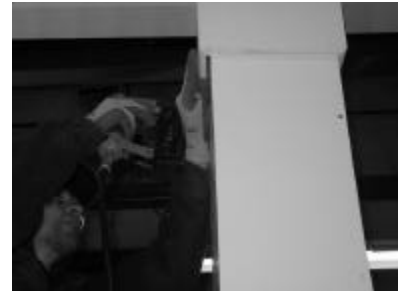
18) Option 1: attach cap to soffit with construction adhesive and toenail to soffit. DO NOT ATTACH cap to column shaft if the cap is flush with soffit (allows expansion.)*
