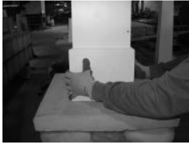
14) Apply adhesive to mitered ends of base moulding (9¼" tall) and assemble around bottom of column shaft.
