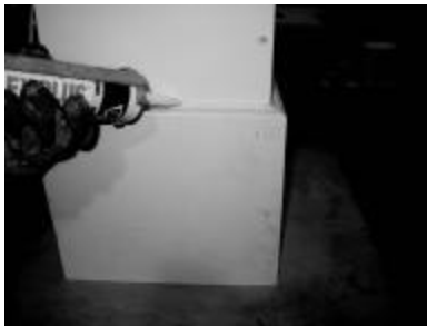
20) Caulk edges of base, cap, and nail or screw holes.
