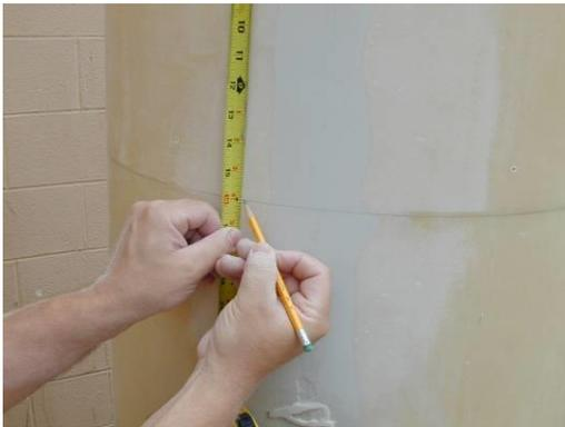
7) Draw a line around the top of the column 16" down from the top of the column. This is the suggested location for the bottom of the neck ring.
