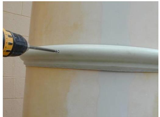
9) Using the 1-3/4" self-drilling screws, install the first neck ring half to the column, lining up the line to the bottom of the neck ring.
