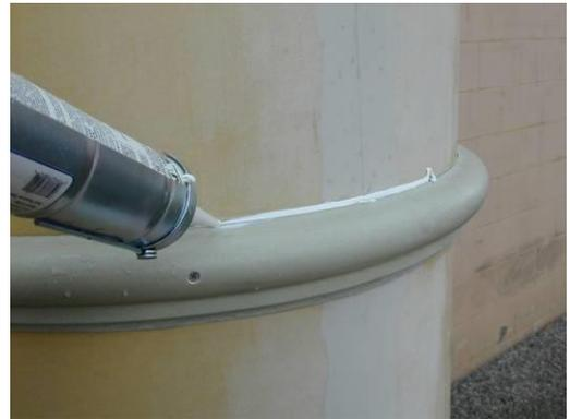
16) Apply a bead of good paintable exterior chalk at the top and bottom joint where the neck ring joins the column. Smooth bead for proper appearance.
