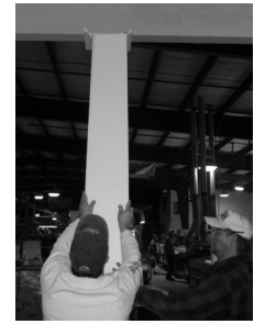
12) Assemble final panel to column using E-Z lock joint. Nail panel to secure in place.
