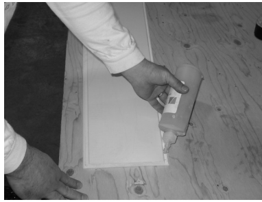
11) Apply adhesive to final panel.
