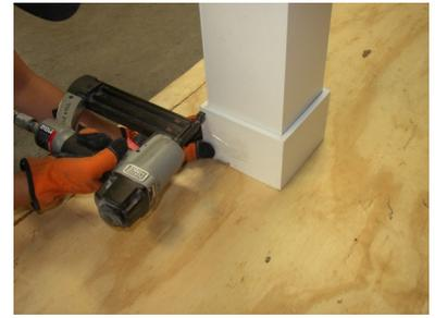
12) Fasten joints on base with pin-nails.
