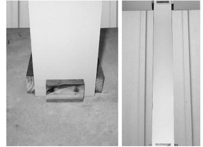
3) If desired, optional blocking (not provided) may be installed around post to center wrap. This is especially helpful when wrapping round or odd sized supports.
